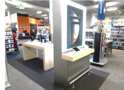
Shelf is not a hazard because a detectable element was added under the shelf
