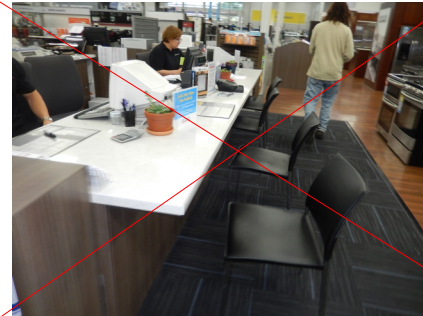
Counter overhangs base for knee/toe clearance and is a hazard – needs an end panel
